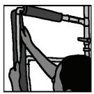
Insulating hot water lines with flexible foam pipe sleeves is cheap and easy and especially important in unheated places.
